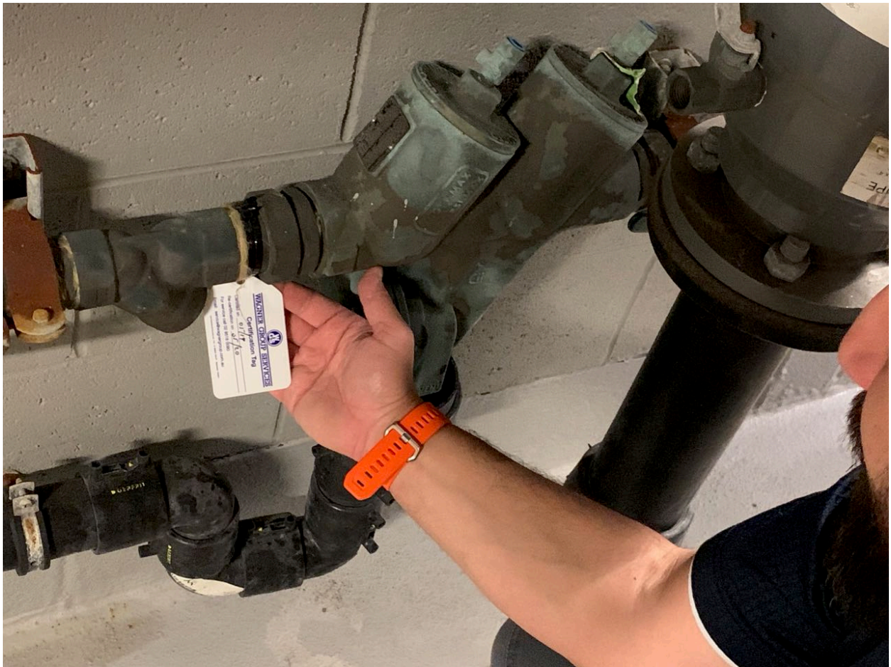
Figure 1. Backflow prevention device with current test tag on the potable water top up feed line.
