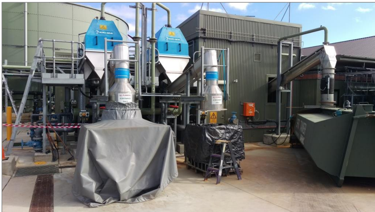
Figure A.11.1 Screening bin currently in use is fully shrouded to prevent waste dispersion and contain odours.
