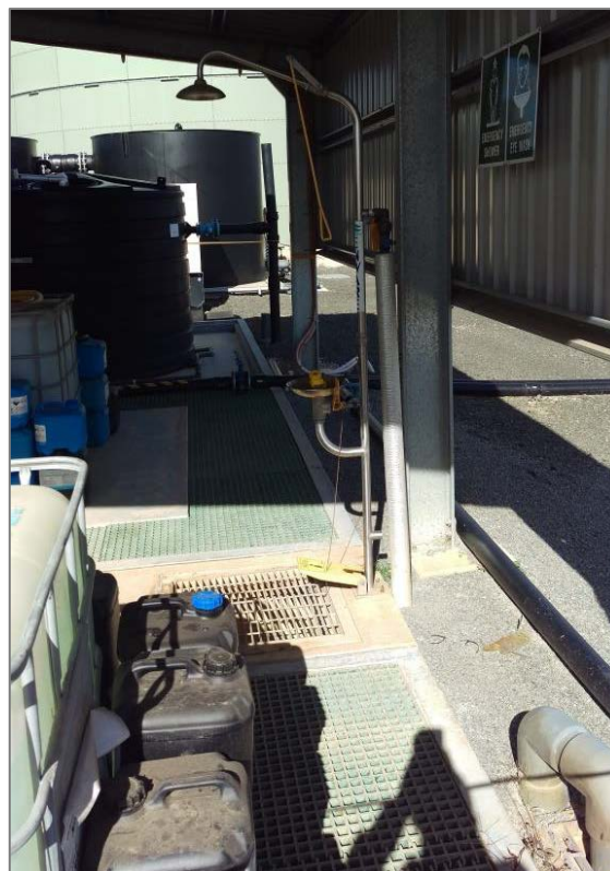
Figure A.11.3 Bunding/containment sumps are in place in the chemical storage area.
