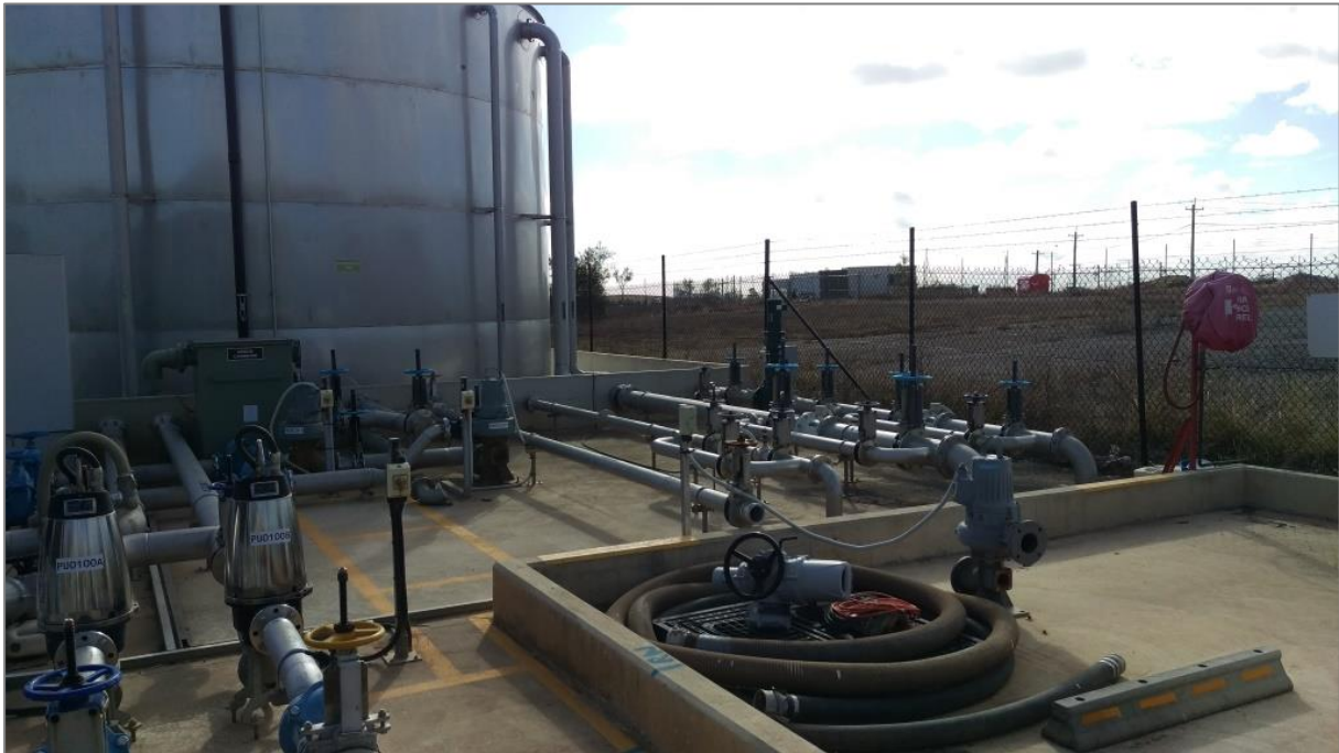
Figure A.11.3 Treatment Plant Inlet Balance Tank is fully bunded.
