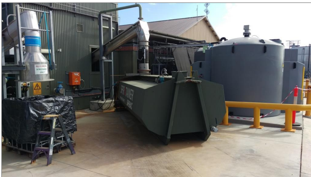
Figure A.11.2 Waste sludge dewatering/biosolids stream is fully enclosed.
