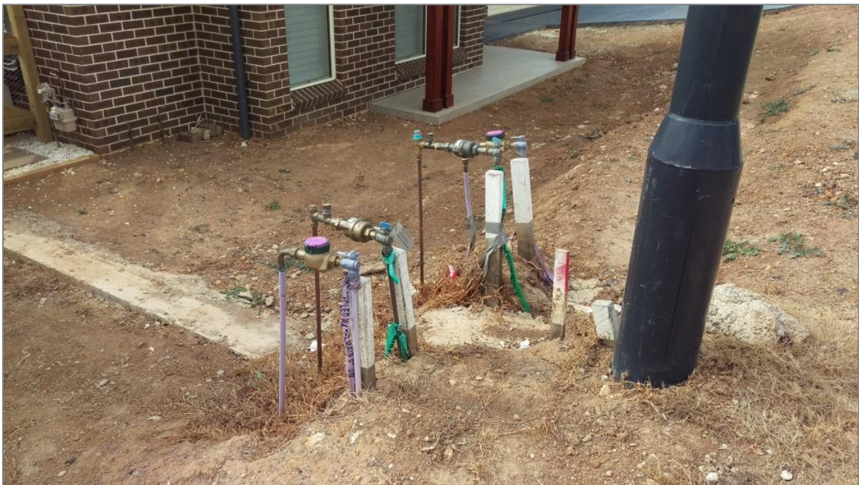
Figure A.3.2 Property connection installations with lilac sleeved risers, marker tape and meter.
