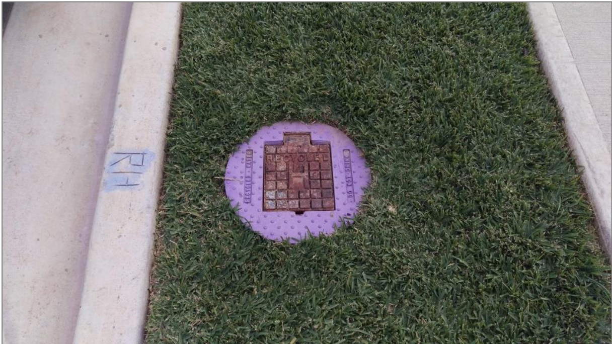
Figure A.3.1 Colour coded valve cover with embossed labelling “RECYCLED WATER; DO NOT DRINK”.
