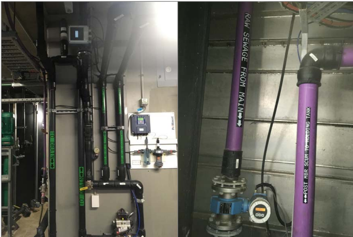
Figure B.3.5 Pipework appropriately labelled and coloured.
