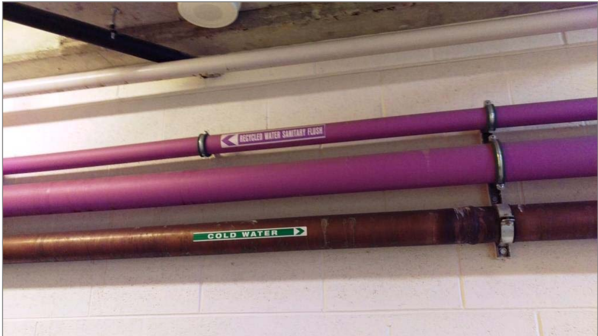
Figure C.2.1 Recycled pipework in basement near the recycled water plant. Note the colour coding and labelling.
