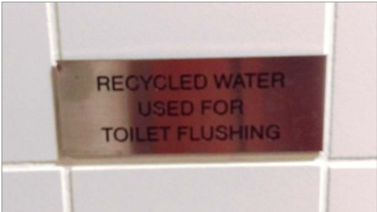
Figure C.2.2 Recycled water labelling in toilet facility.
