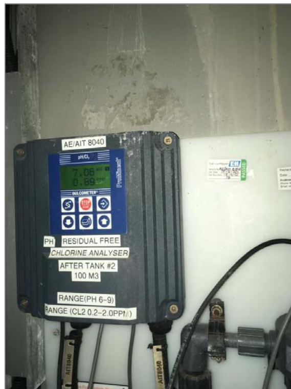
Figure C.1.1 pH and residual free chlorine analyser – Tank No: 2.
