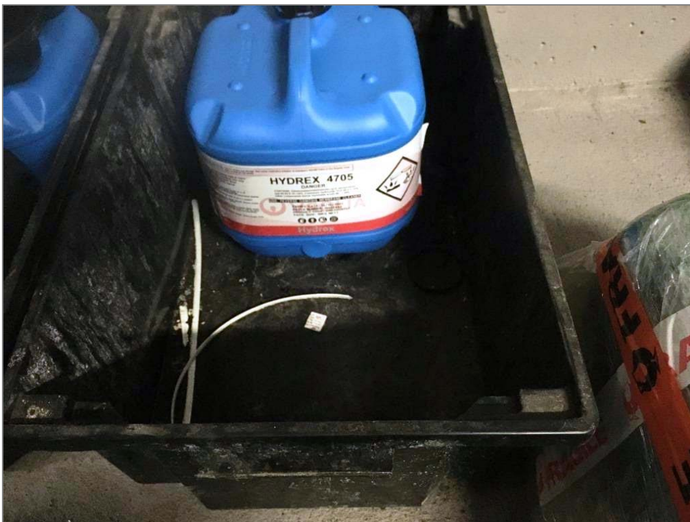
Figure B.3.4 Chemical container stored within an empty tub (bundling).
