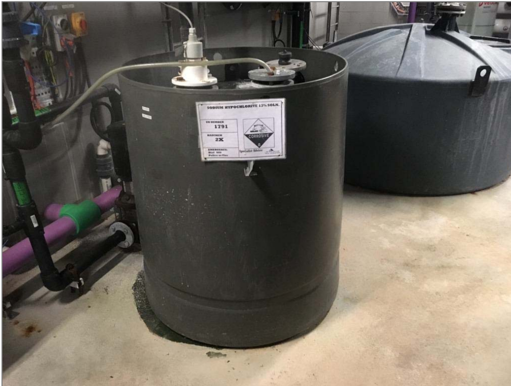
Figure B.3.3 Self-bunded chemical storage (inner storage tank contained within an outer tank). Note clear chemical signage.
